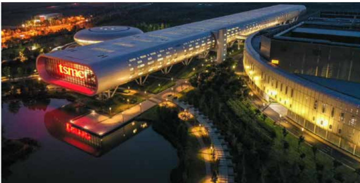
Taiwan Semiconductor Manufacturing Facility
